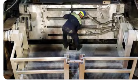
Picture 7: Works on the new platform. Picture courtesy of Acerinox Europa.
