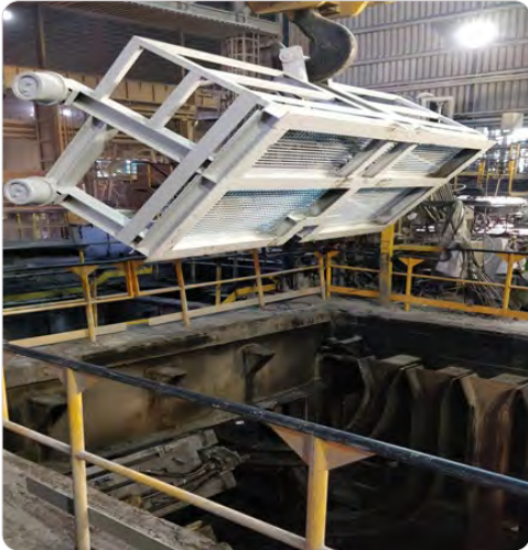
Picture 5: Lifting of new platform. Picture courtesy of Acerinox Europa.
