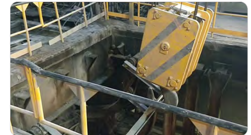
Picture 4: Installation of new platform. Picture courtesy of Acerinox Europa.
