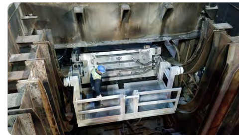
Picture 3: New platform mounted. Picture courtesy of Acerinox Europa.
